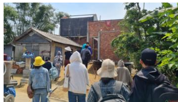
Fig.1. Building safe house for beneficiaries
