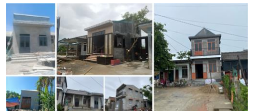
Fig.6. 07 completed houses in Q.A & Q.T
