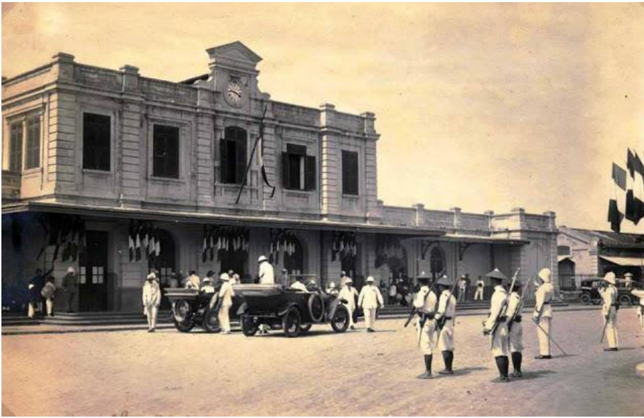
Figure 1: Hue Station, Built in 1902 and Still in Use Today
